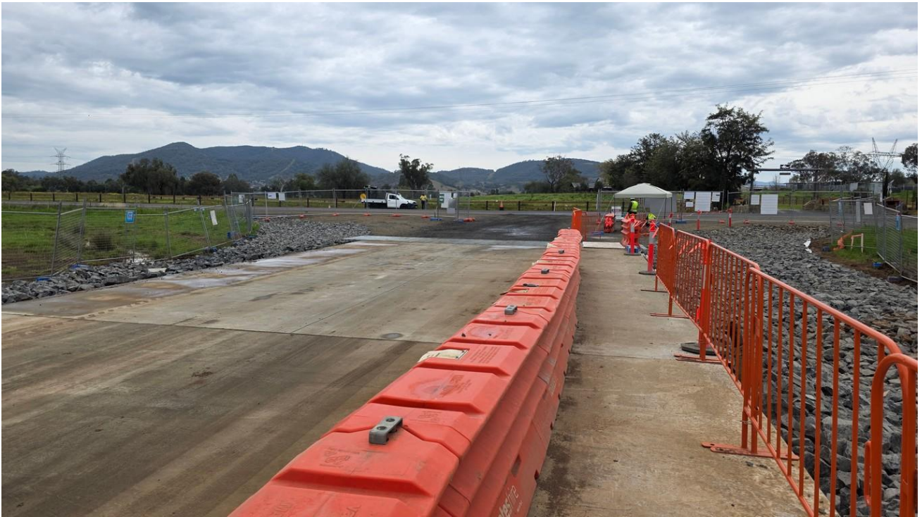
Photo B10(c)(ii)-3: Safety barriers installed to separate pedestrian pathways from vehicle access routes
