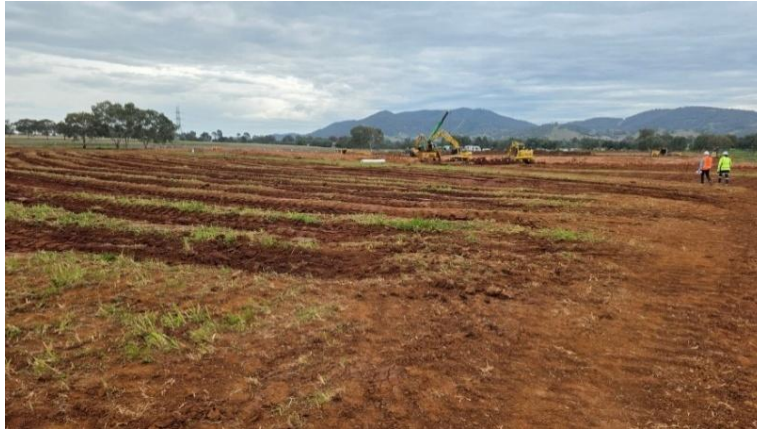
Photo B12-1: Early works involving BESS preparation, with further excavation occurring for constructing bioretention basin
