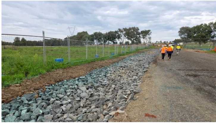
Photo B28-4: Rock-lined perimeter drain and the newly built culvert crossing
