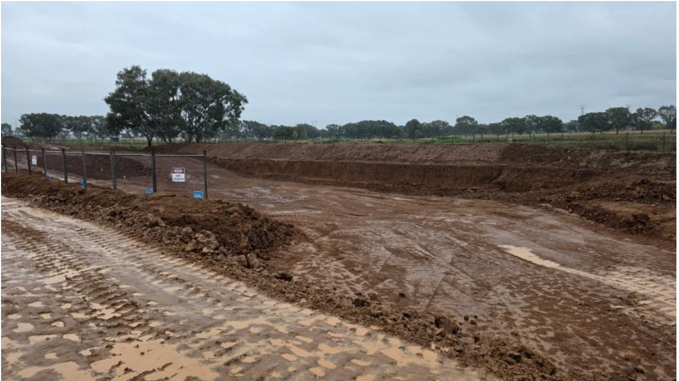
Photo B11-4: Topsoil segregated from excavated materials
