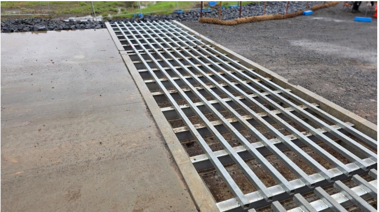
Photo B9-1: Shaker grid installed near site access point adjoining culvert
