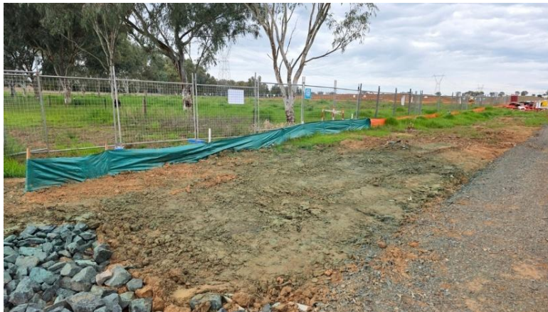
Photo B28-5: Erosion and sediment control measures in place, including a silt fence near a gravel access road and open grassy area.
