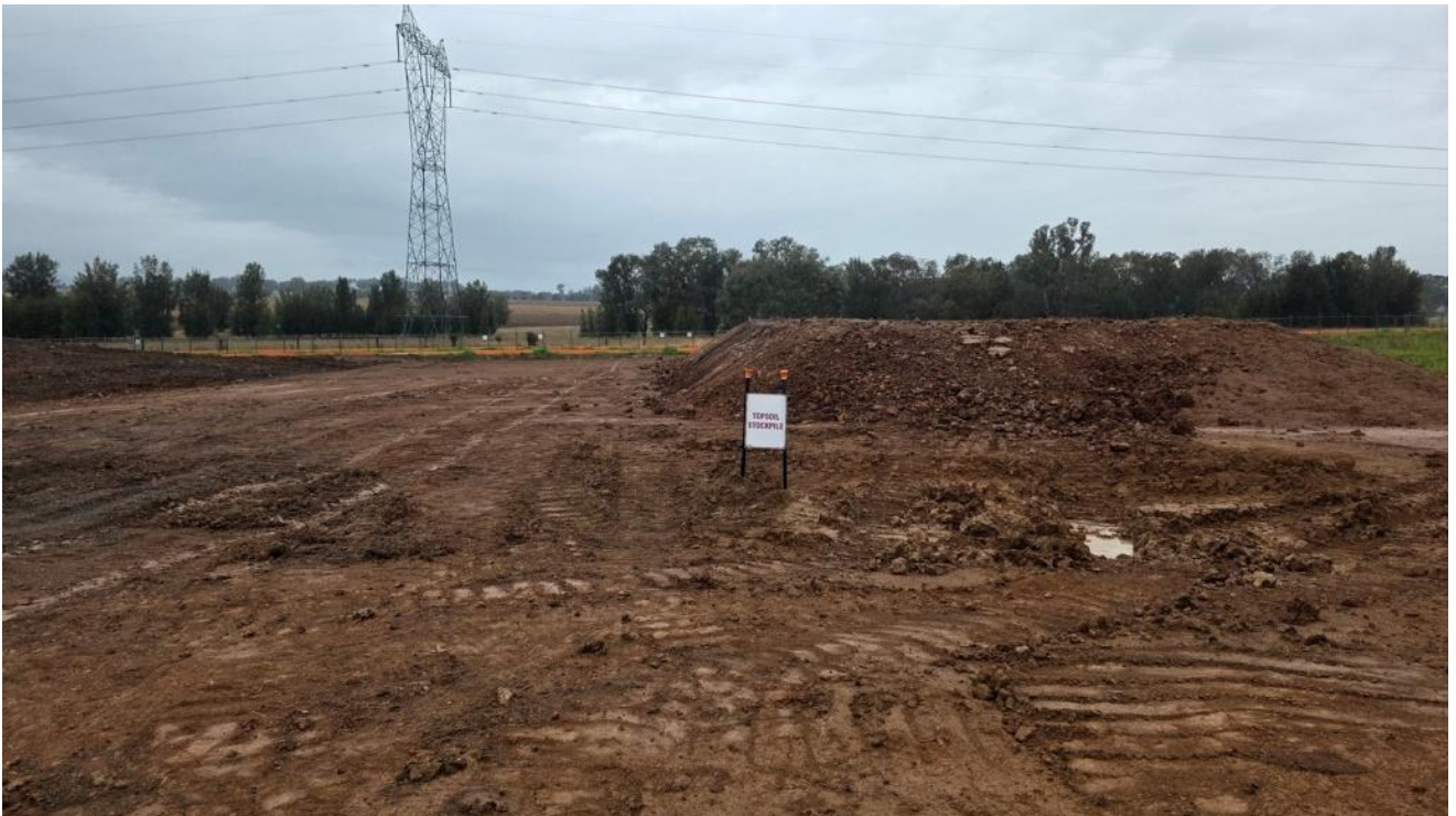
Photo B11-4: Topsoil segregated from excavated materials
