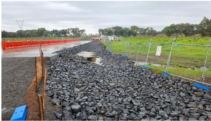
Photo B28-5: Erosion and sediment control measures in place, including a silt fence near a gravel access road and open grassy area.
